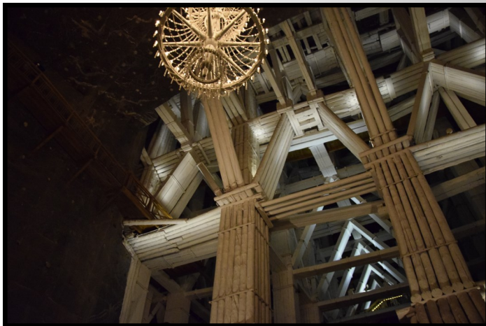
Mine shaft reinforcement in the mine (fot.35.)
