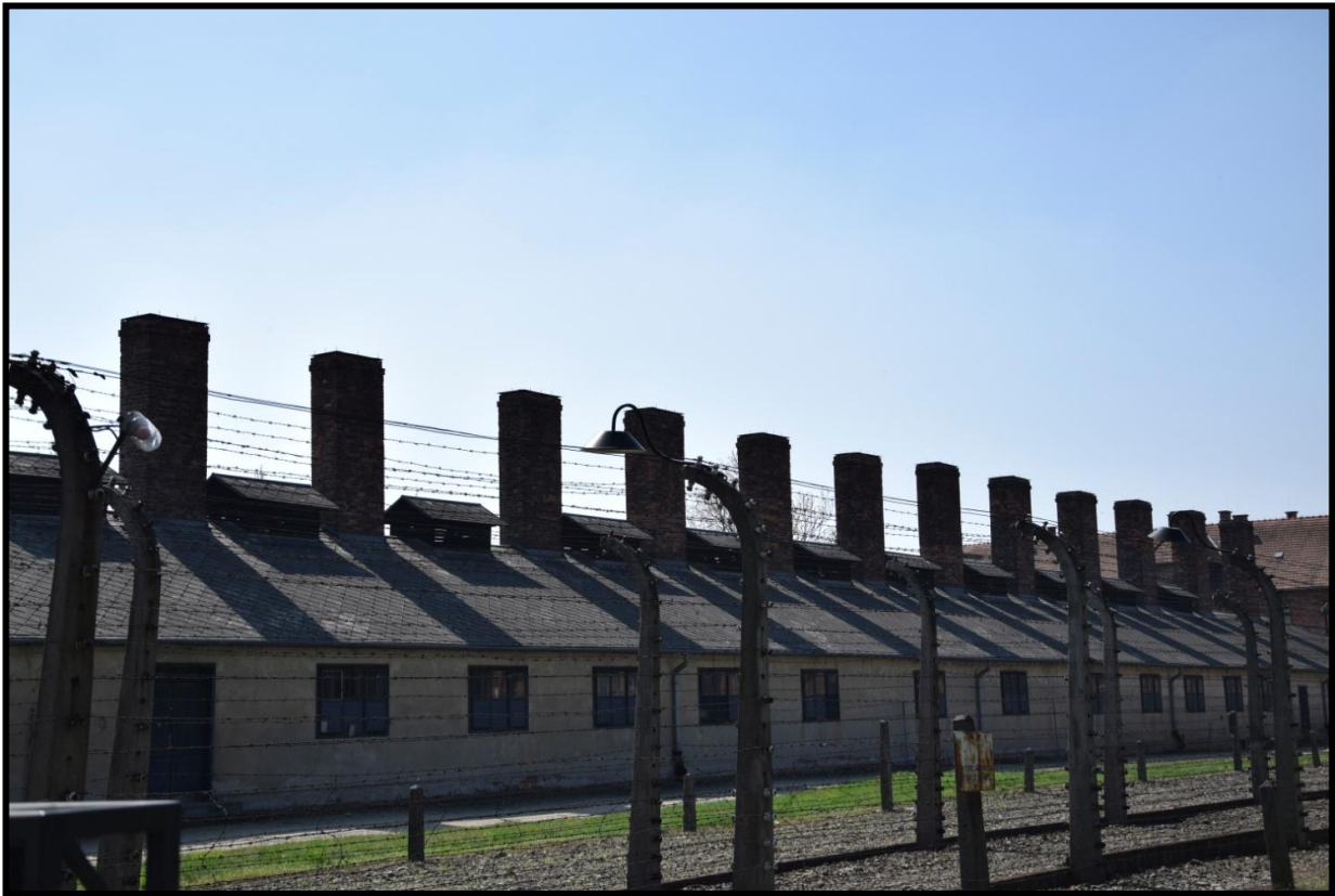
Auschwitz camp buildings (fot.21.)
