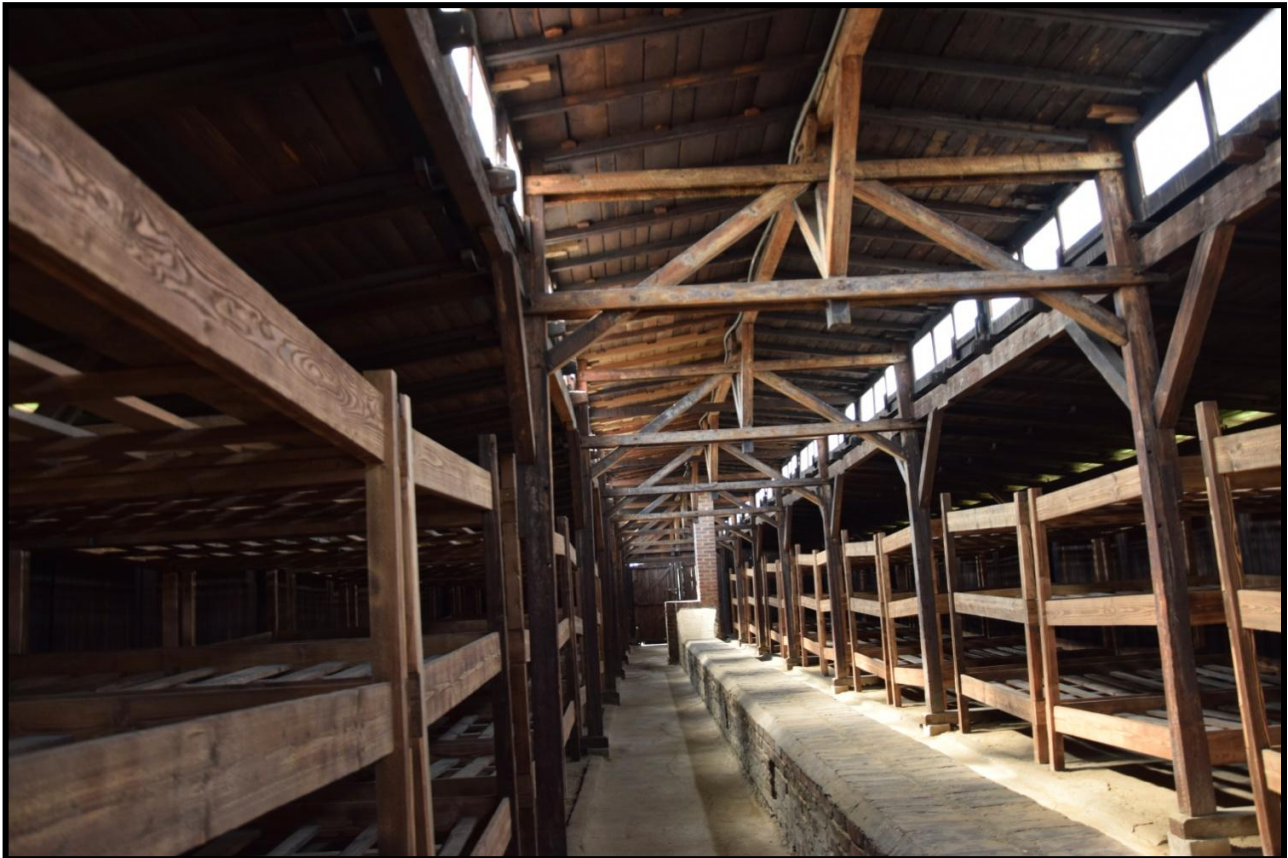
Barrack's interior in Birkenau (fot. 25)
