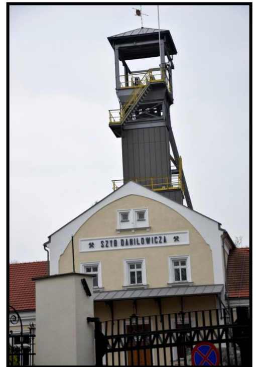
Entrance to the mine (fot.34.)
