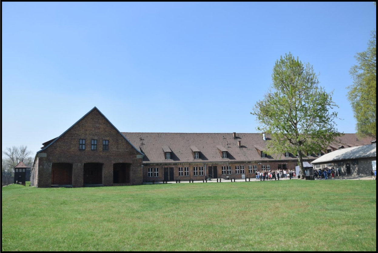
Auschwitz camp buildings (fot.22.)
